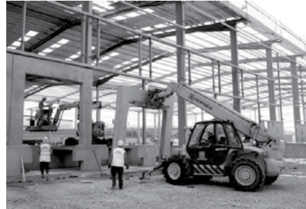
Photograph 2.1 Framed construction with prefabricated bathroom and service pods.
