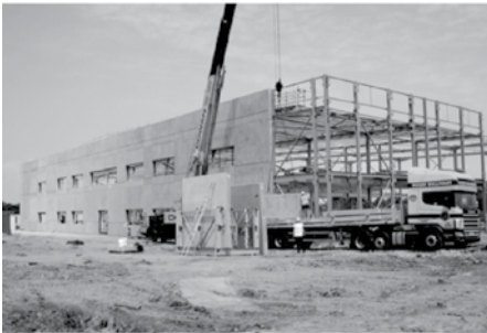
Photograph 2.1 Framed construction with prefabricated bathroom and service pods.
