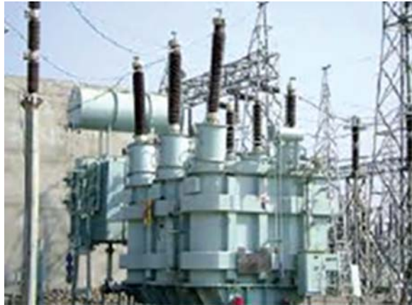
Figure 2.4 Large oil filled transformer.
