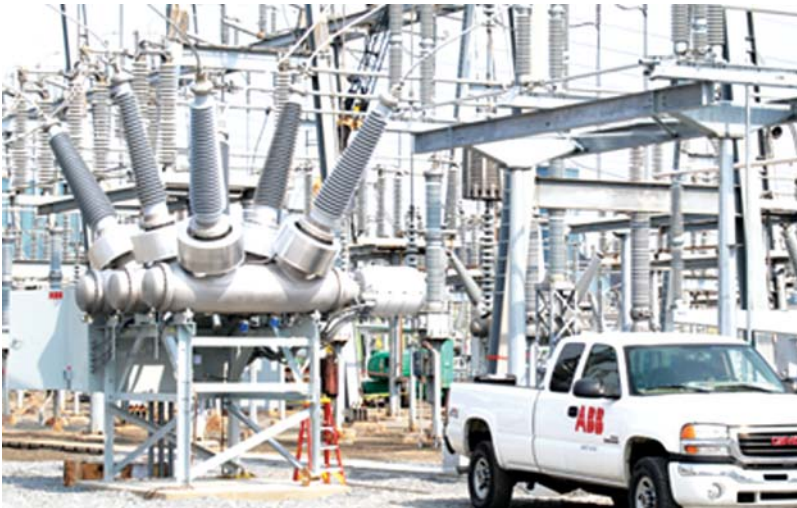
Figure 2.5 245 kV circuit breaker.
