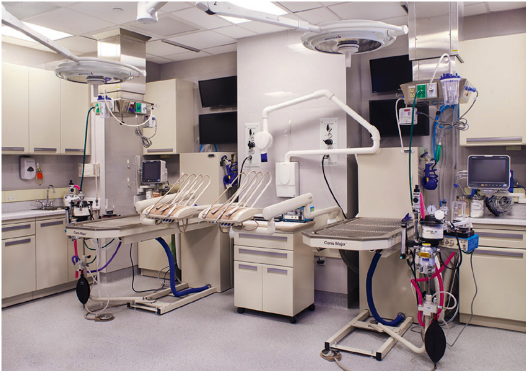
Figure 1.25 Wall-mounted X-ray generator to service two treatment tables. Source: Courtesy of The Animal Medical Center, in New York City.
