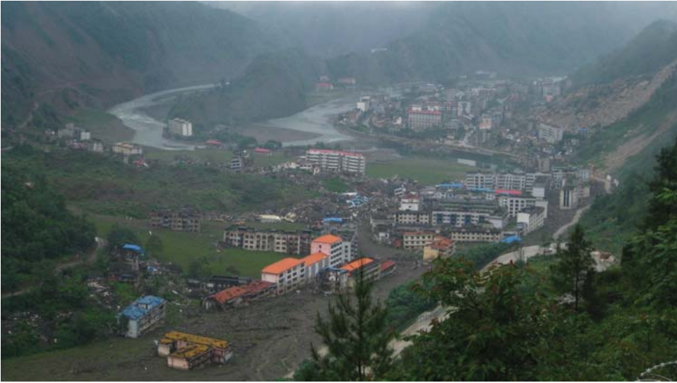
Figure 1.8 The earthquake hazard cascade in Beichuan, Sichuan province, China, after the Ms 8 Wenchuan earthquake in 2008. Buildings collapsed or were severely damaged due to the strong ground shaking. The shaking also triggered several landslides that invaded the town. A large landslide dam upstream of the town had to be artificially breached, sending floodwaters and sediment through parts of the city. Monsoon rains mobilized more landslide debris from hillslopes months after the earthquake, triggering a series of debris flows that caused massive aggradation of up to several meters. (Tim Davies)
