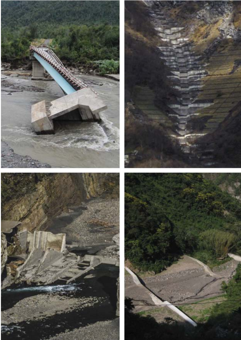
Figure 1.10 Pulsed sediment transport can damage infrastructure. Dealing with the problem requires understanding of sediment delivery mechanisms, sediment volumes, duration, and spatial reach. Top left: Bridge destroyed by a lahar, Chile. Top right: Cascade of check-dams and sediment retention basins in a mountain stream near Nikko, Japan. Lower left: Collapsed sediment retention basin in a steep mountain watershed, Taiwan. Bottom right: A series of check-dams filled with sediment, Taiwan (all photos by Oliver Korup).
