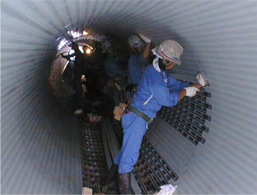
**Photo 1.4:** A composite pipe renovation method by using evenly-spaced steel frames and long PVC plates to fabricate interlinings before grout injection
