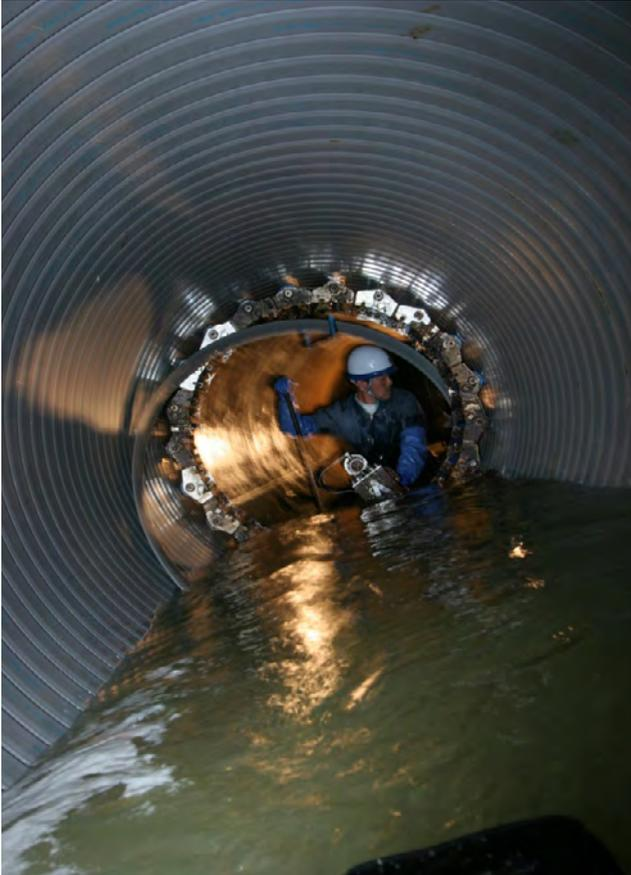
**Photo 1.3:** An ageing sewer during renovation construction by using the SPR method
