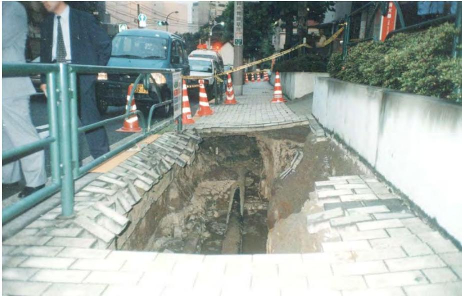
**Photo 1.1:** Road cave-in caused by the collapse of a sewer main (Tokyo)
