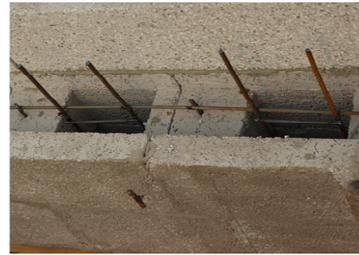
Fig.7 Fix vertical steel meshes
