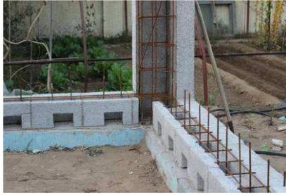
(a)construct the first row blocks and lay the first piece of horizontal steel mesh
