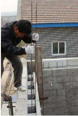
Fig.6 Inset vertical steel mesh into cavity
