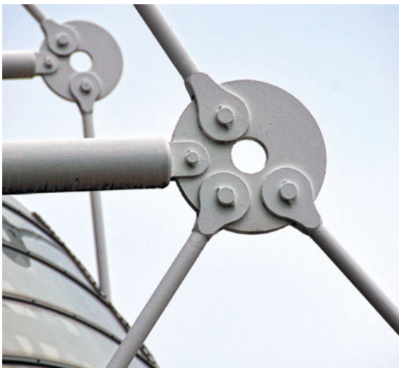
High Tech detailing such as explored in the Centre Pompidou needed to address the use of force-differentiated systems. The use of exposed tension systems had to that point not formed a dominant theme in architecture. The geometric resolution of multiple forces through a point, as explored in the Centre Pompidou, was to become an important design focus in the development of AESS systems.
