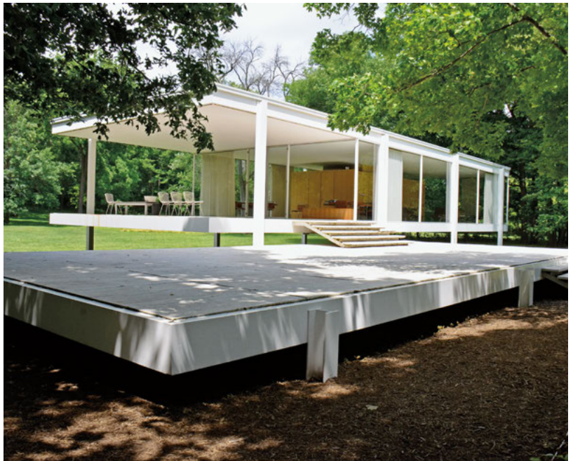
The iconic Farnsworth House in Plano, IL, USA, designed by Ludwig Mies van der Rohe, 1945–1951, makes use of simple hot-rolled shapes (channel, wide-flange and angle). The connections were welded to keep the detailing very clean and somewhat "mysterious".
