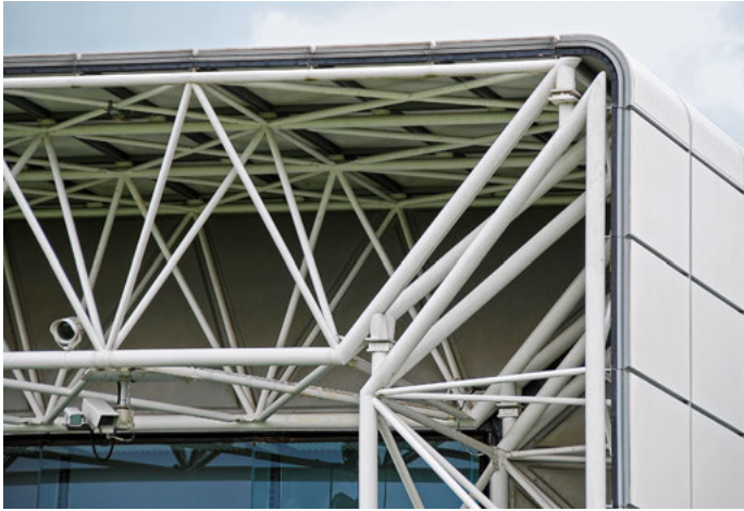
The Sainsbury Centre for Visual Arts in Norwich, England, designed by Foster + Partners, 1977, demonstrates the very specific use of structural sections and connection detailing that distinguishes High Tech from the International Style. Hot-rolled tubular steel was quite new at the time of construction of this project, necessitating new approaches to fabrication and connection design.
