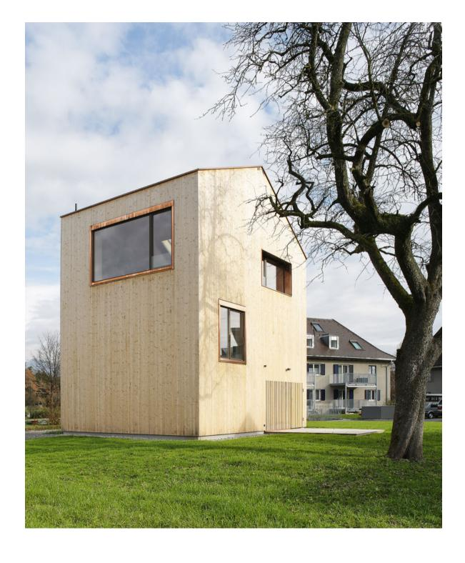
The rear-ventilated facade of this three-storey house consists of rough-sawn fir wood boards that can be fitted when still moist, thanks to a vertical tongue and groove joint. The prefabricated wooden substructure meant that the entire assembly, including the fitting-out of the interior with birch plywood paneling, could be completed in a day and a half—allowing the building costs to be substantially reduced.
