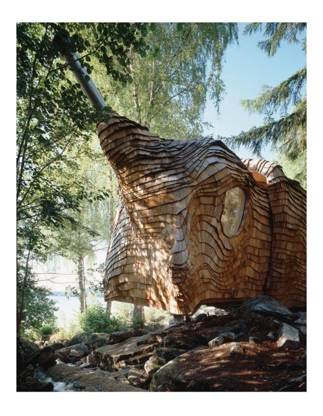
The organic structure of this house is ideally adapted to its natural  $% \left\{ 1,2,\ldots ,n\right\}$ forest setting. A section of the house is mounted on castors, allowing it to be slid in and out like a drawer. The roofing shingles, a traditional material used for roofs in Sweden, are made from Western Red Cedar, a wood that requires no further maintenance.
