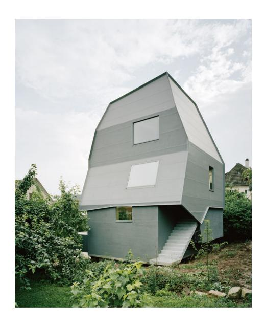
This building constructed of solid timber elements was prefabricated in modules, assembled on site, and completely covered with a roof foil of synthetic rubber. The house consists of a total of 136 individual elements. Before being assembled, rebates were made in them for
