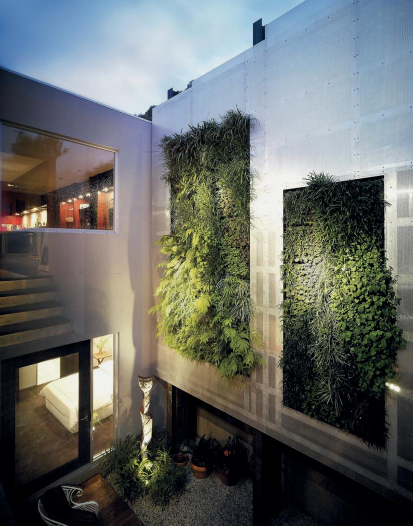
The colour, transparency and texture of the wall are different at different times of the day. The spaces for the planned planting modules for the two Fytowalls were cut out of the aluminium, and containers made from plastic-coated, watertight plywood with an overall surface area of 10.5  $\rm m^2$  were fitted into the gaps to house the wall planting systems and all installations. The outer edges of the planting modules are flush with the aluminium surface.
