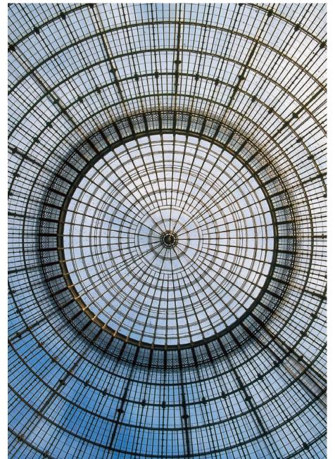
ducing the load-bearing framework that supported the glass panes.
