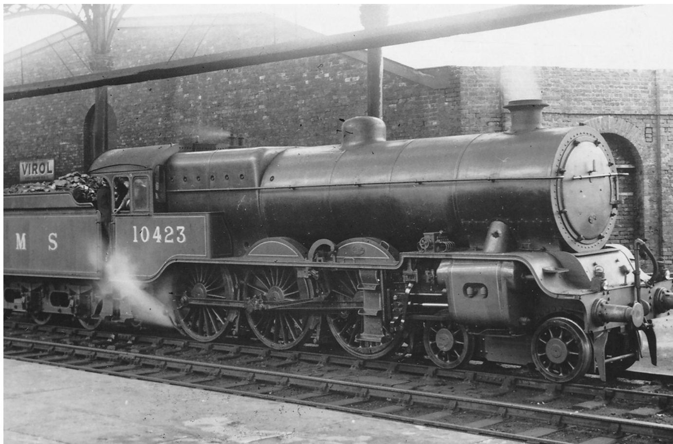
George Hughes' 'Dreadnought' 4-6-0 10423, built in 1921 to the 1919 rebuilding design of the 1908 four-cylinder L&Y 4-6-0, c1925. It was withdrawn in 1948. (R.K. Blencowe / MLS Collections)
