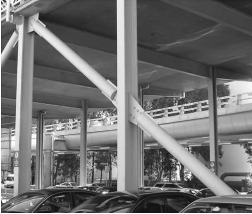
Figure 3. Statically-loaded steel frame, braced with diagonal hollow sections.
