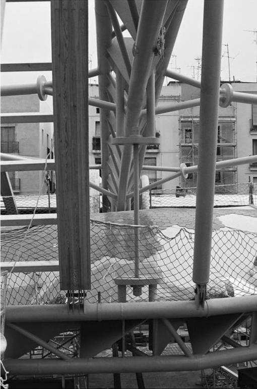
Figure 5. Connection of the hangers to the steel beams.
