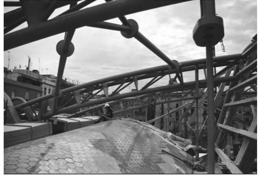
Figure 7. General view of the bracing.
