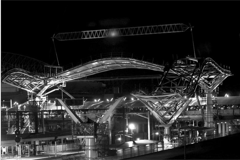
Figure 1. Erecting the spine truss.
