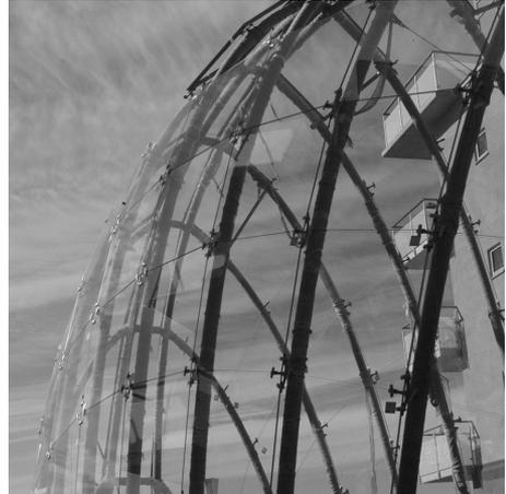
Figure 16. Close-up of the glass panels and the supporting steel structure during installation.
