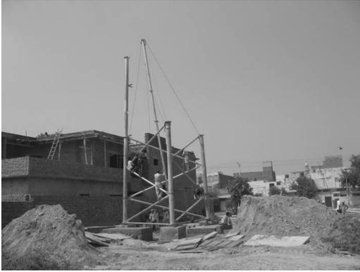
Figure 13. Erection of a tower of tubular elements in Pakistan using simple methods.
