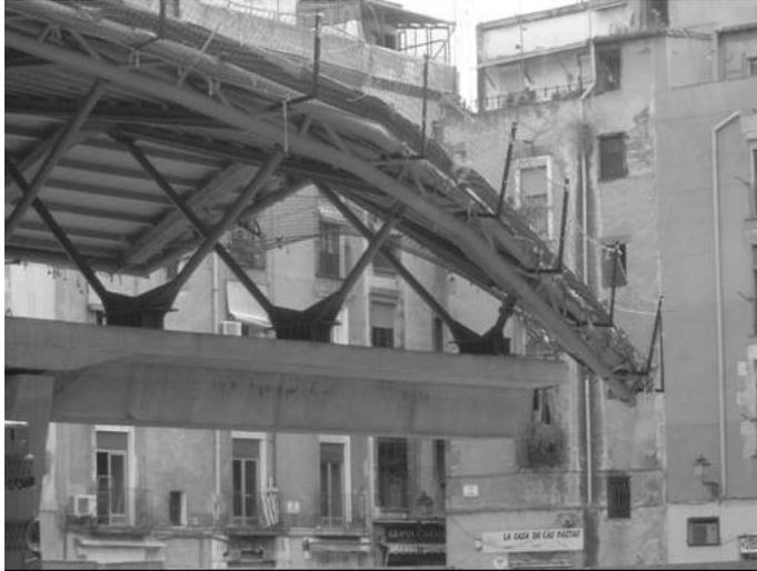
Figure 14. Concrete cantilever, tubular steel props and beam, and wooden arches.
