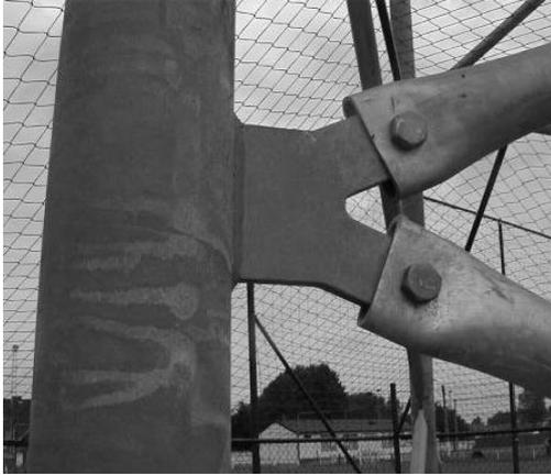
Figure 9. New joint between diagonal and leg, both circular tubes. BASE, Belgium.
