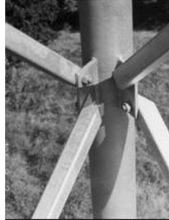
Figure 11. Eccentric joint between diagonal and leg, PANNON, Hungary.
