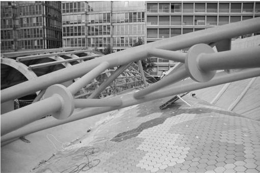
Figure 6. Local view of the bracing.
