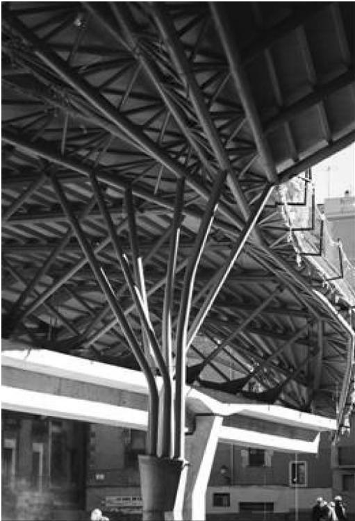
Figure 11. Tubular steel beams. South facade.
