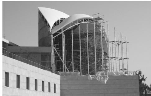
Figure 12. During installation of the roofs the *central body* was temporarily supported by scaffolding.
