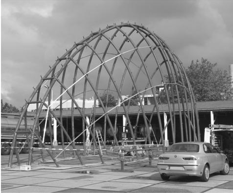
Figure 15. Test assembly of the steel structure in Delft.
