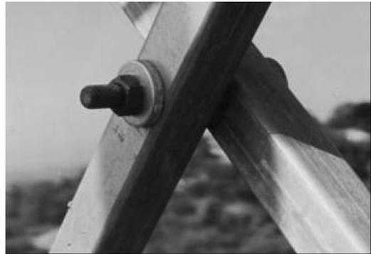
Figure 12. Joint in the intersection between cross bracing, PANNON, Hungary.
