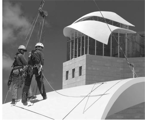
Figure 11. Hoisting of one of the roof shell wings.
