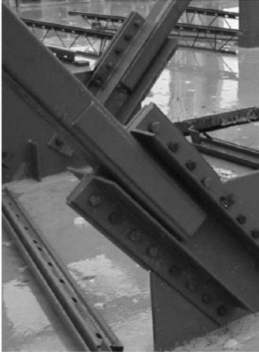
Figure 11. Fabricated square HSS gusset connection for seismic application. (Photo courtesy of Pierre Gignac, Canam Group, Canada).
