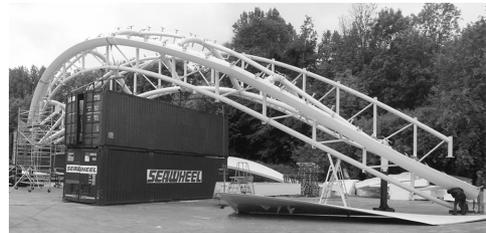
Figure 9. Test assembly of the *central body* (spanning 30 m) in Lelystad at Holland Composites.
