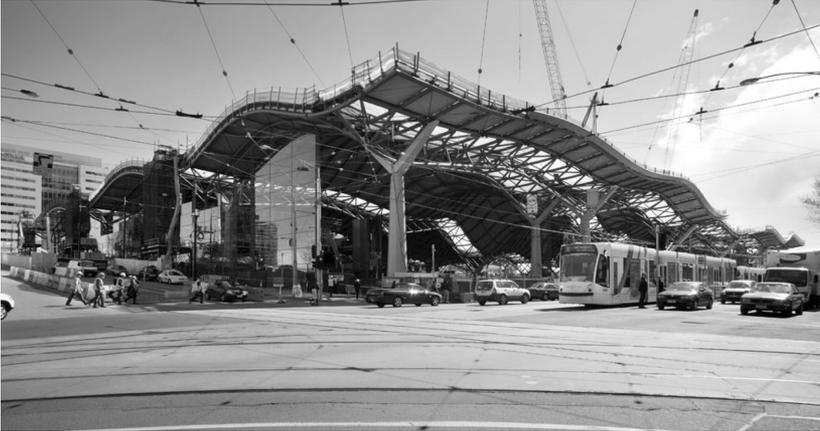
Figure 5. Tree columns supporting the roof.
