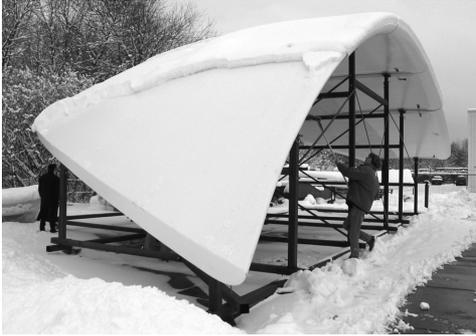
Figure 10. GRP roof segment assembled on a temporary steel structure at Holland Composites in March 2005.
