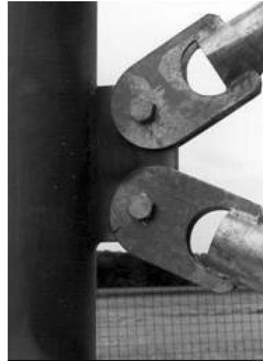
Figure 7. Traditional joint between diagonal and legs, both circular tubes (ONE, Austria).
