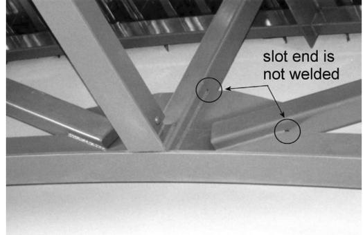
Figure 4. Square HSS diagonals with slotted ends, in a roof truss.
