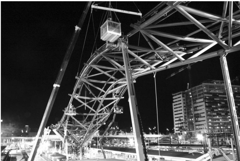
Figure 2. Insertion of an arch section.
