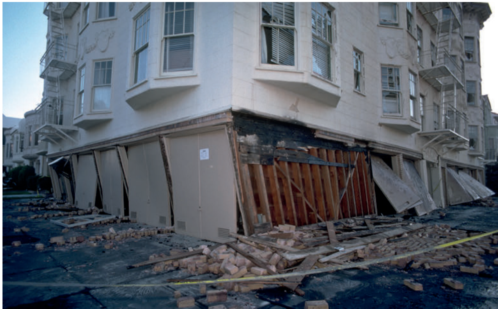
1.1 Example of structural damage in a building with inadequate shear walls at the garage level. Loma Prieta earthquake, San Francisco USA, 1989
