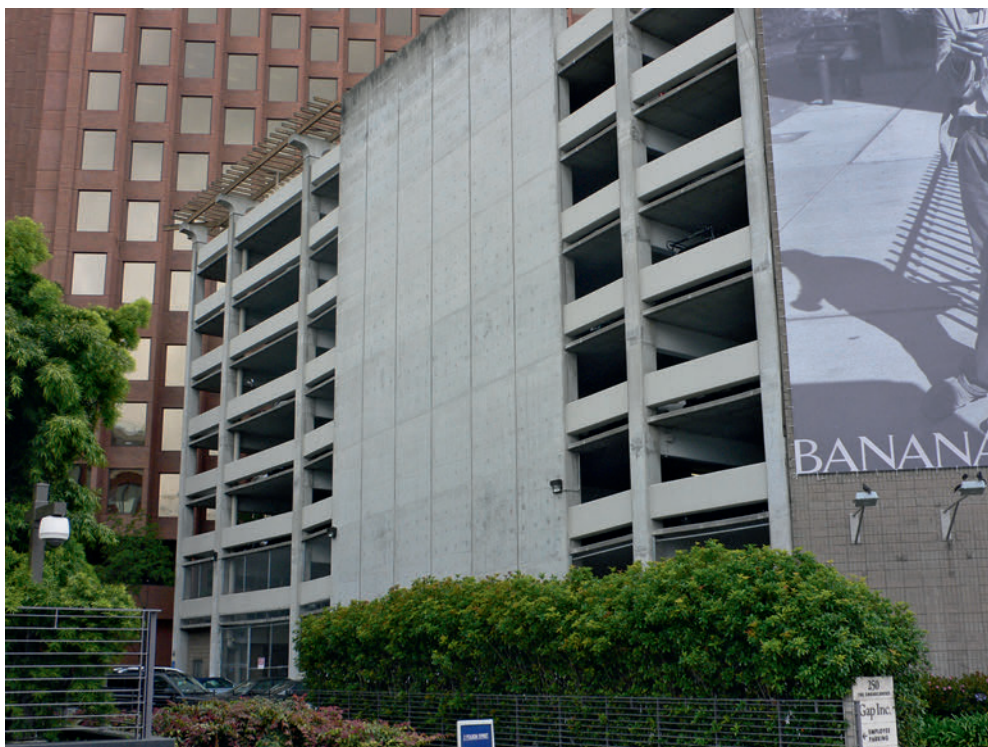
1.4a Example of a type of structural system: shear wall
