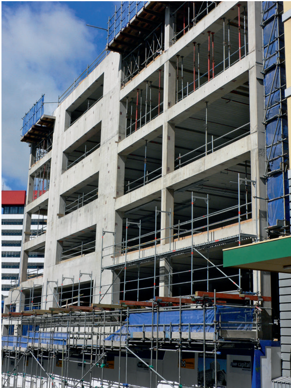
1.4b Example of a type of structural system: single-bay moment frame
