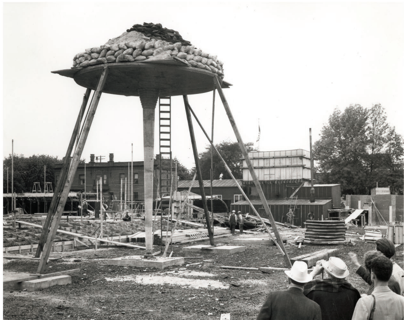
Figure 0.1 Frank Lloyd Wright observing the full-scale mock-up of his column design. Frank Lloyd Wright, S.C. Johnson Wax Administration Building (Racine, WI, USA) 1937.
