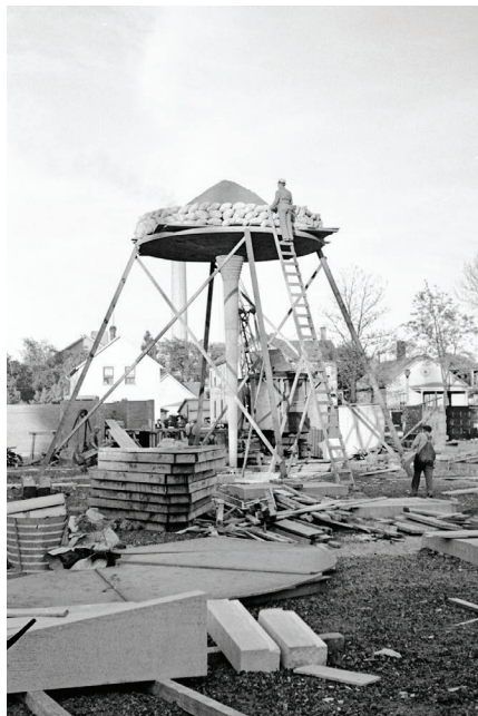
Figure 0.2 Contractor Ben Wiltscheck climbs a ladder to determine how much more sand can be added, 1937. Frank Lloyd Wright, S.C. Johnson Wax Administration Building (Racine, WI, USA) 1937.
