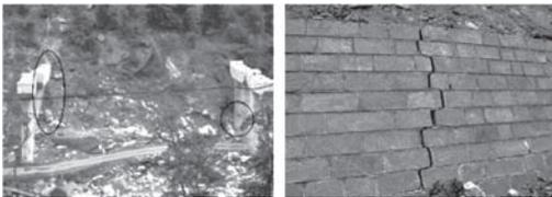
Figure 21. Structural damage after talus slide: damaged bridge piers (left) and crack in retaining wall (right) (Liu 2011).
