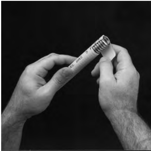
Fig. 1.3 Strip back the cover
