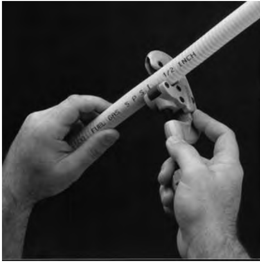
Fig. 1.2 Cut the TracPipe to length
