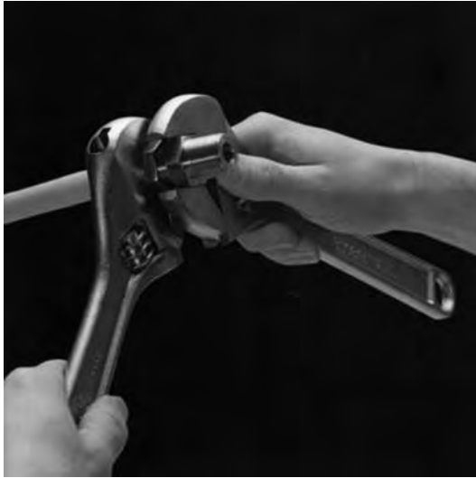
Fig. 1.5 Complete final connection
