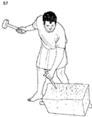
57 A stone-mason rough dressing a facing stone with a punch or point.
