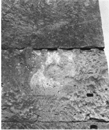
38 A block of tufa with the traces of the sockets for the wedges that were used in cutting it up (Pompeii VIII, 5, 30).
