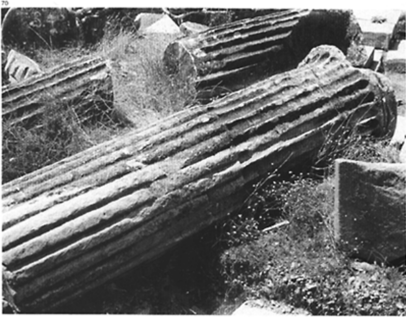
70 Unfinished column from the Temple of Euromos (Caria). The fluting was prepared by an axial groove indicating the depth to be reached.
