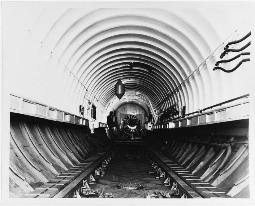
Figure 1.2 I-400, or I-401 (Japanese Submarine 1944) interior of the aircraft hangar, showing tracks for rolling planes out (October 14, 1945)
