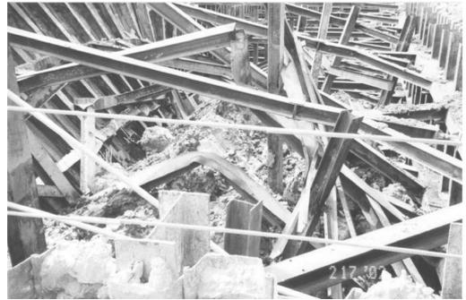
Figure 22. The failed section of the excavation for the Central Services Tunnel, showing the failed base just above the jet grout slab and the north wall rotated inwards.
