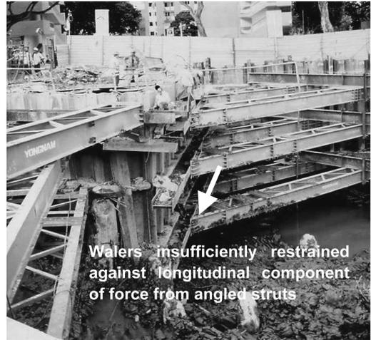
Figure 24. The walers in this photograph had moved longitudinally, allowing the wall to deflect by over 600 mm.
