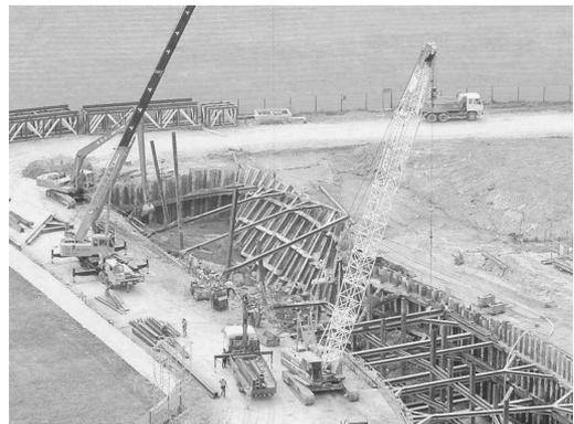
Figure 23. The failed excavation during recovery. Note the kingposts in the failed section, some of which had been pushed upwards by 3 m, and the rotational failure of the retaining wall.
