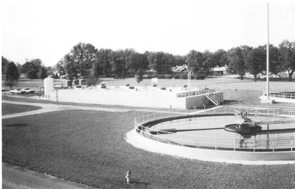
FIGURE 8. 7.5 MGD UNOX® System at Speedway, Indiana. (Courtesy of Union Carbide Corporation.)
