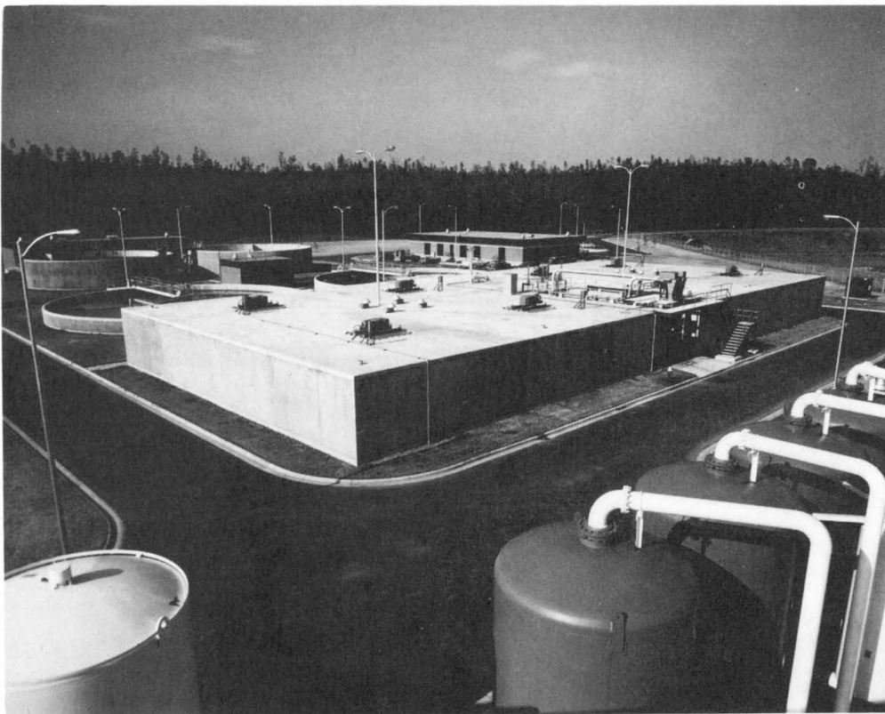
FIGURE 9. 8 MGD UNOX ® System at Morganton, North Carolina. (Courtesy of Union Carbide Corporation.)
