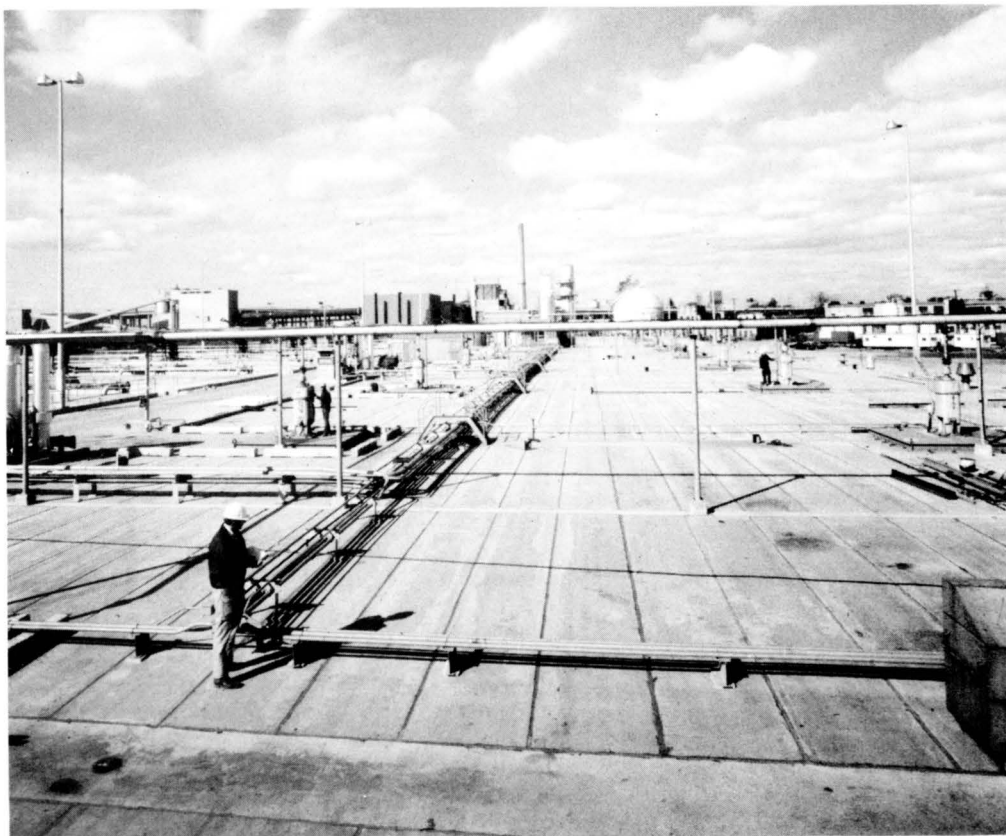
FIGURE 5. Overall view of 300 MGD UNOX ® System at Detroit, Michigan with 180 ton/day cryogenic oxygen plant and 900 ton liquid oxygen storage tank in the background. (Courtesy of Union Carbide Corporation.)
