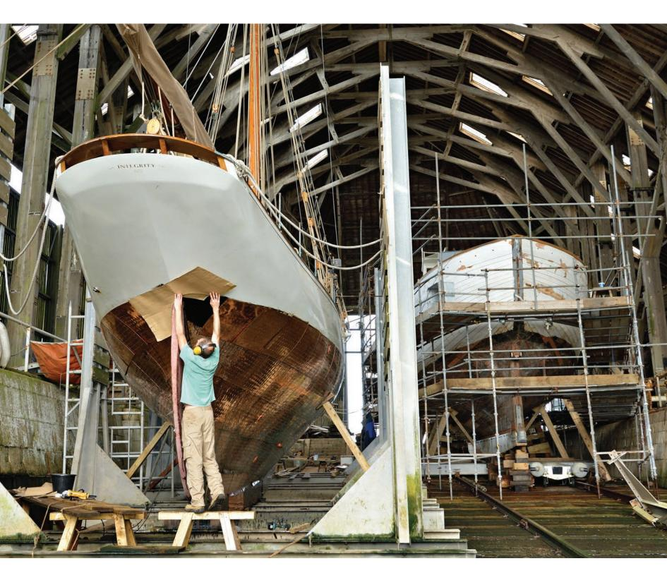
building pilot cutters. As working vessels, the essential feature of these crafts was speed. The pilot's job was to guide a larger ship safely into harbour – and there were usually more pilots than ships requiring help, so it was a case of the first one on board getting the job.
