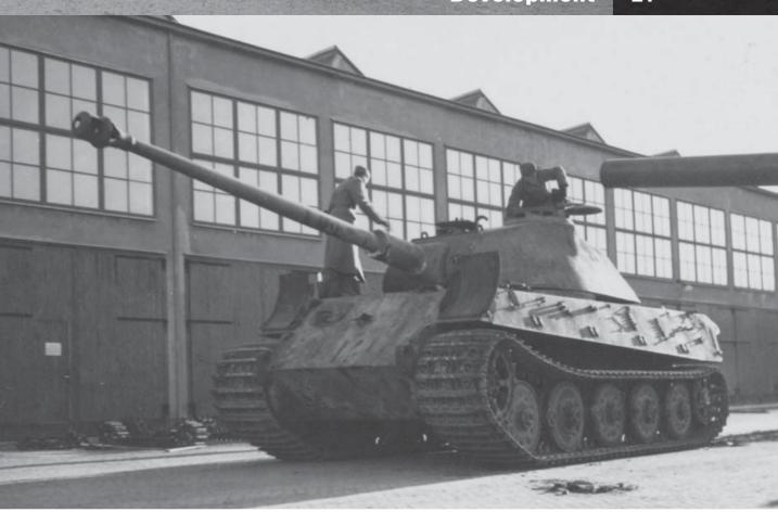
The armour plates of the new tank were sloped, creating a tank similar in appearance to the PzKpfw V Panther. The thickness of the frontal armour was significantly increased (from 100 to 150mm) but the side and rear plates of the hull remained at 80mm, but with an improved slope.
