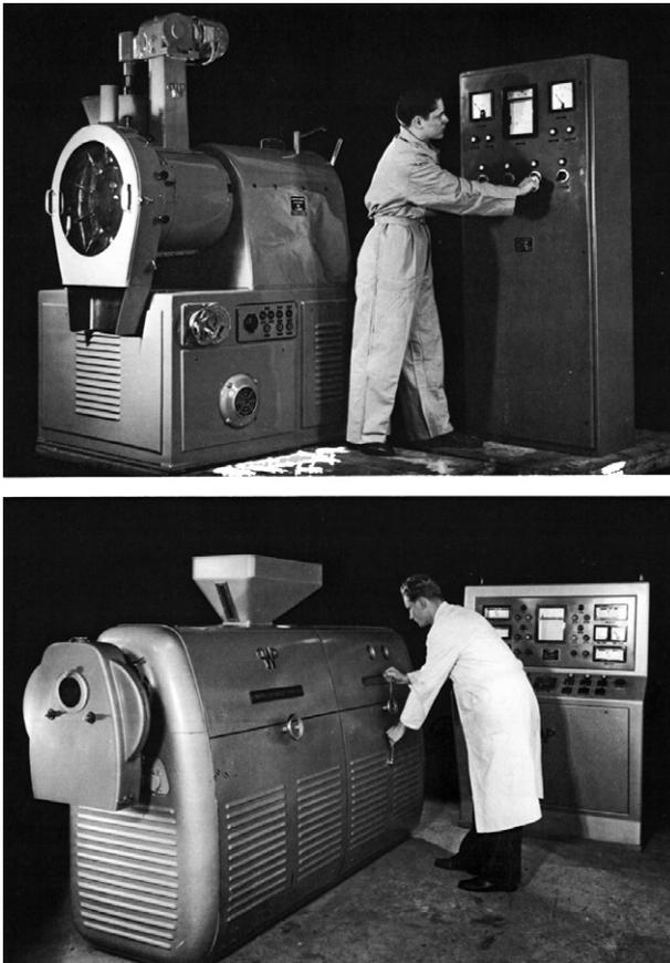
**Figure 1.7** Werner & Pfleiderer’s ZSK machine from the 1950s. Original figure caption: “In the 1950s WP, together with major chemical companies, made a significant contribution to the burgeoning age of plastics. The top figure shows a plasticizing unit for producing flexible PVC, the bottom figure the first twin-screw extruder for compounding plastic pallets”
