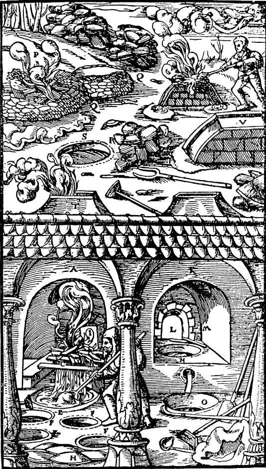
Figure 1.1 Sixteenth century furnaces for smelting lead ore
