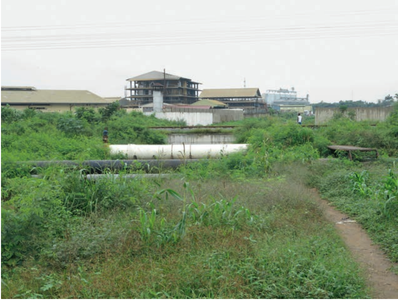
Plate 2. Trunk sewer lines across Chemu Lagoon from defunct sewage pumping station, 2014 (Photo by Eva Egensteiner)
