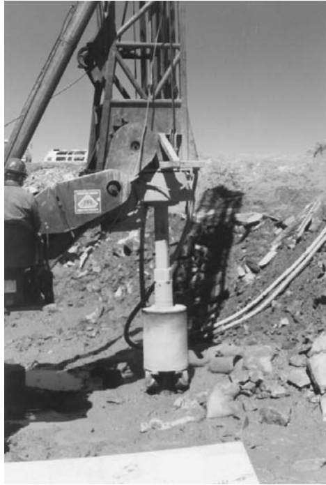
FIGURE 2.1 Caisson rig with a rock bit.
