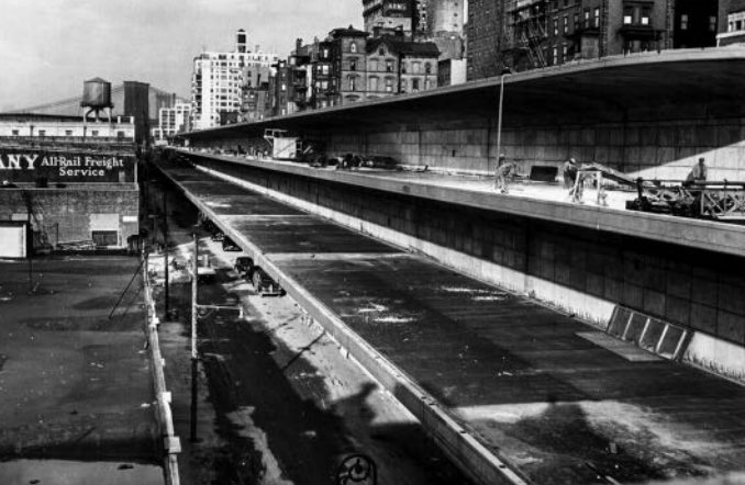
Figure 1-4. Construction of the Brooklyn-Queens Expressway's triple cantilever section with the Promenade on top was underway in 1948. The Promenade would be completed to its full length in 1951, and the expressway would open in 1954, dramatically changing the edge of Brooklyn Heights and cutting off Montague Street's access to the waterfront. (J. Brunelli / Brooklyn Historical Society.)
