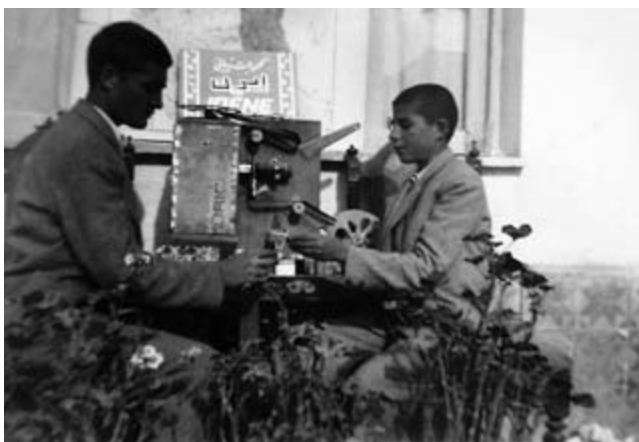
13 Building a 35mm film projector. My cousin, Alireza Naficy, eighteen years old (left), and his classmate, Hodayun Shahriari (right), with the 35mm projector they built in 1955 in the backyard of Shahriari's house in Isfahan. Still courtesy of Alireza Naficy
