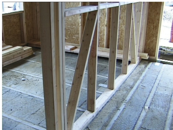
Figure 2.1 This photograph shows both off-site construction (the timber frame) and on-site construction (the beam and block floor)
